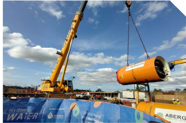
Austral Leppington Wastewater Stage 3, NSW. SUMIT role: NEC4 commercial management. Image: Abergeldie.
